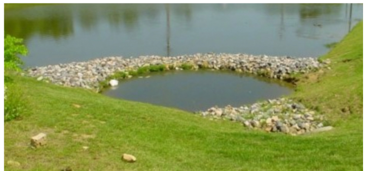
Stock photo of a sediment forebay. Source: Internet
